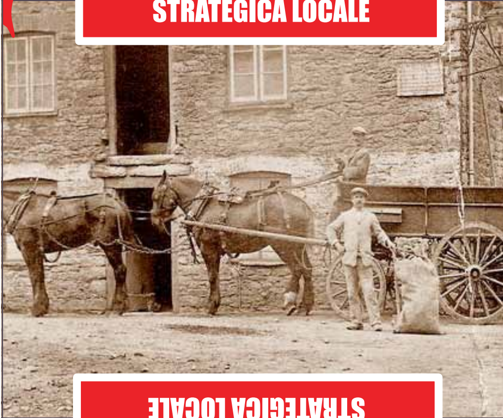
The last working mill in Toines before its closure. Photo - Toines Image Bank and Rural Archive
